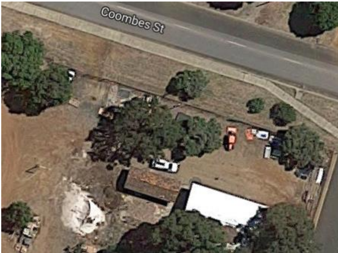
Storage shed at the Former Depot
