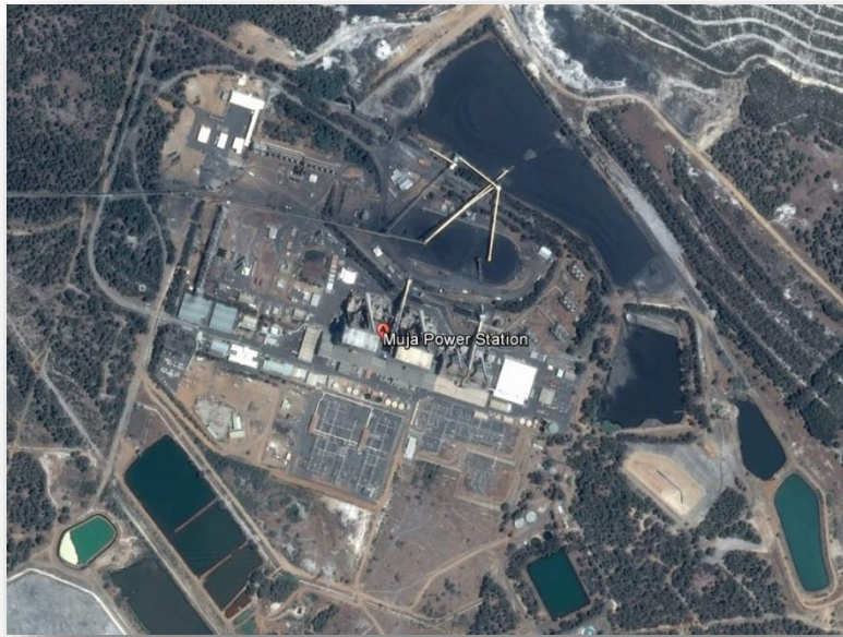
Figure 9 - Muja Power Station (Source: Google Earth)
