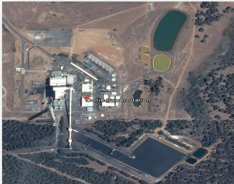
Figure 10 - Collie Power Station (Source: Google Earth)
