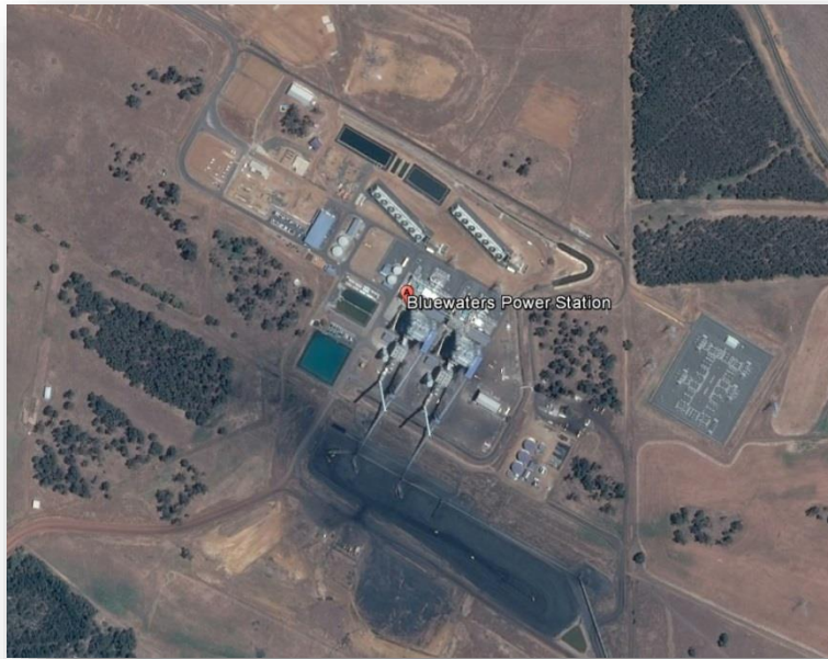
Figure 11 - Bluewaters Power Station (Source: Google Earth)
