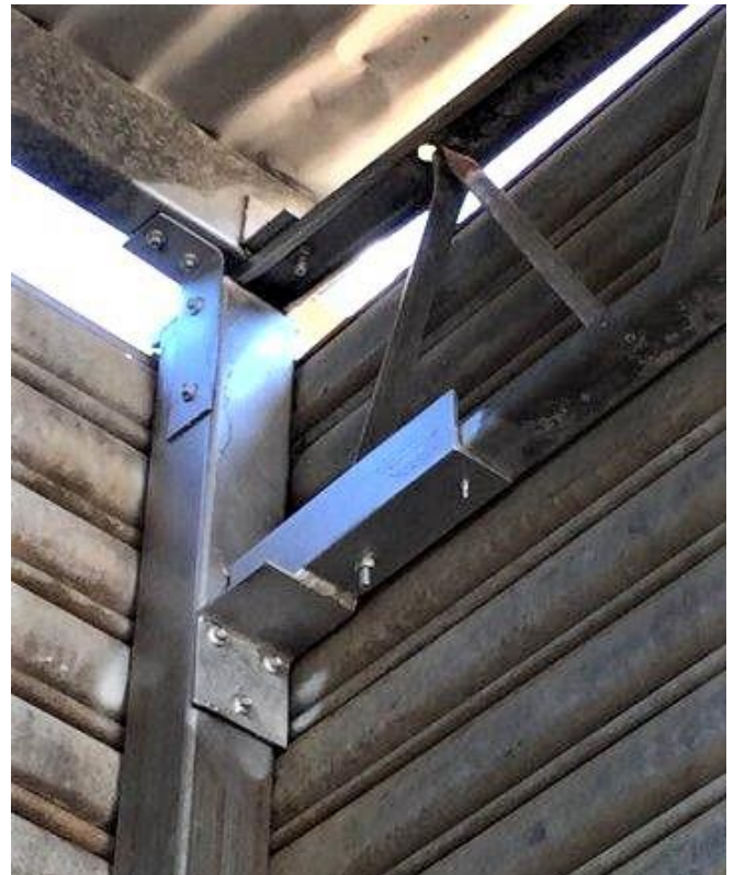
N/W corner post - truss
