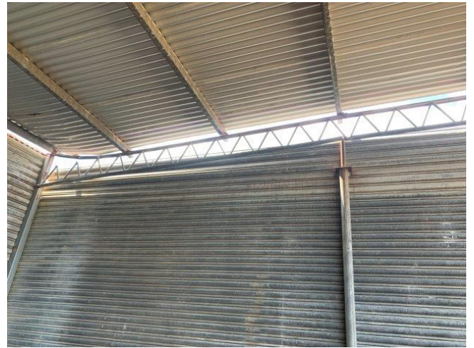
North end – damaged truss
