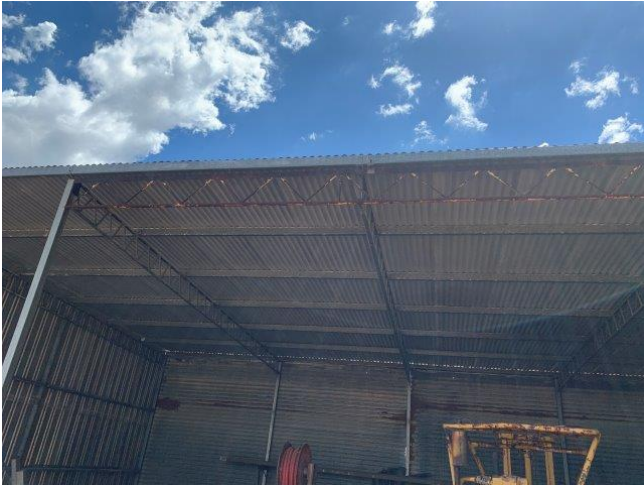
Pipe truss over 2 bays
