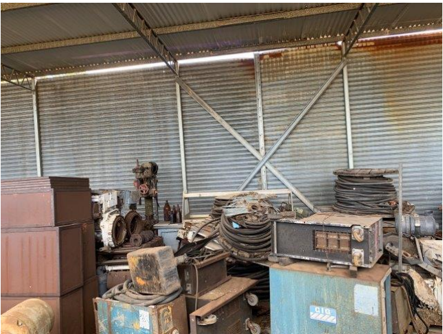
West wall – centre strap bracing
