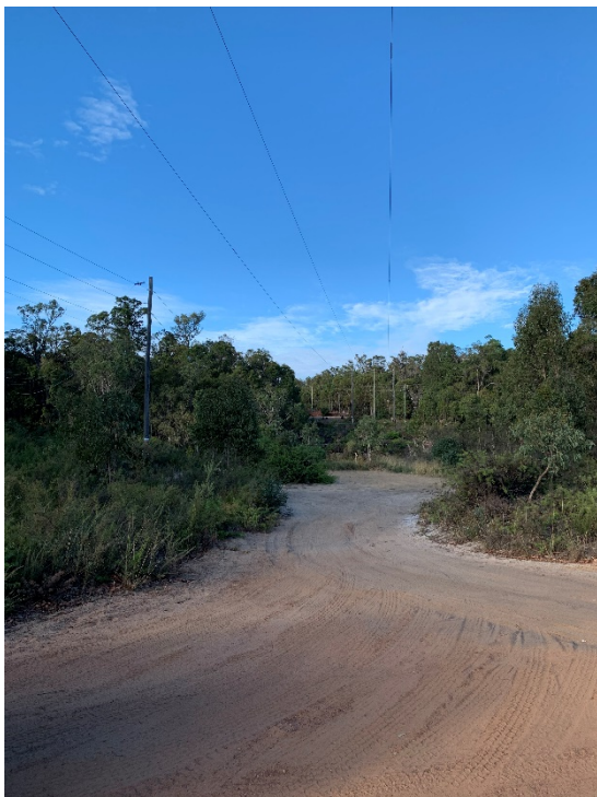
Image 1: Existing Western Power Aerial Cabling
