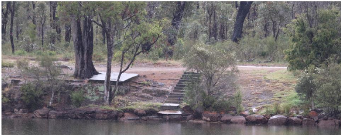
Figure 4: Site 1: Minningup Pool Concrete Stairs from Shore Coastal Technical Note
