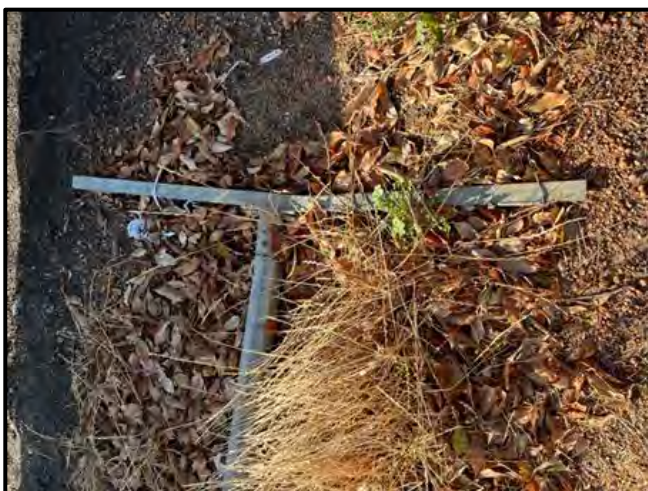
Image 08 – Pole 5355 Pole Tip with Bent Crossarm
