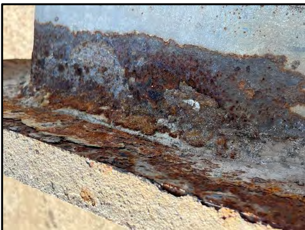
Image 04 – Pole 5252 Corroded Base Section
