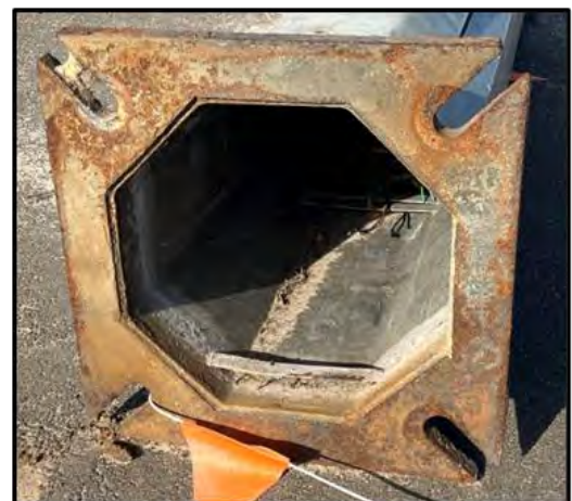
Image 05 – Pole 5252 Corroded Base Plate
