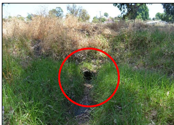
Plate 8: Stormwater discharge point and minor gully erosion
