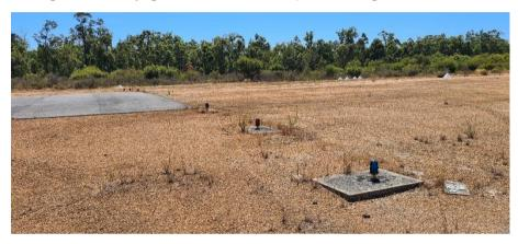
Figure 22 Runway end lights - threshold 28
