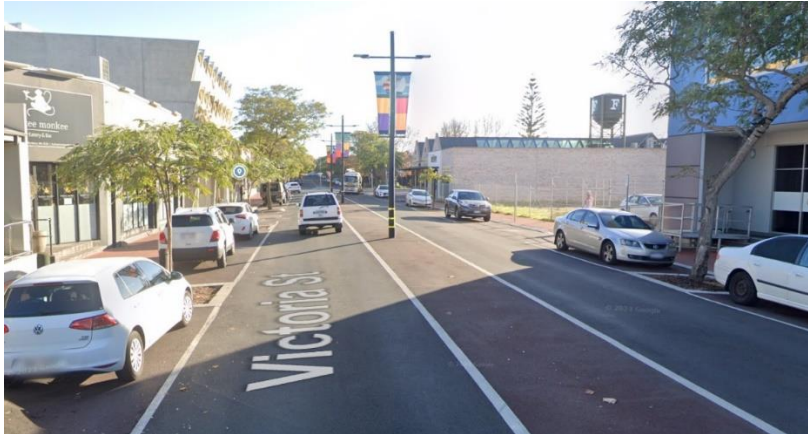
Figure 2 – Example of finished project (Victoria Street, Bunbury)
