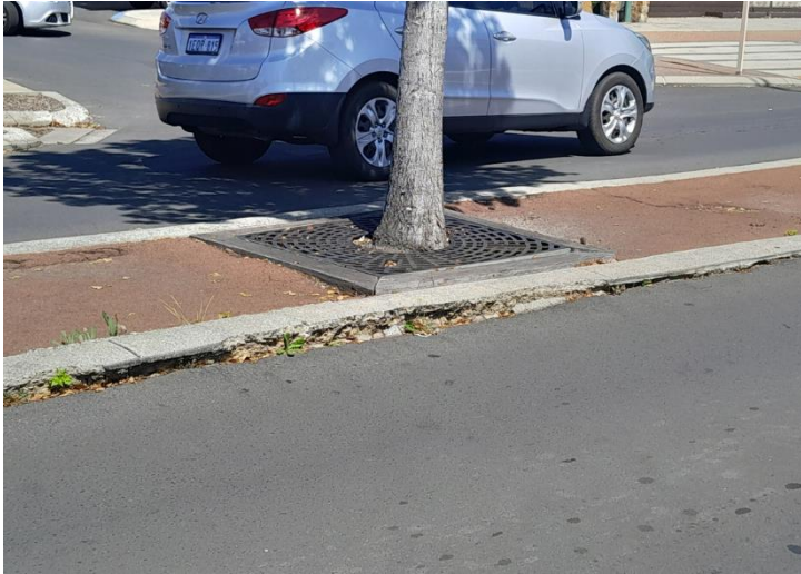
Figure 1 – Example of lifting flush kerb
